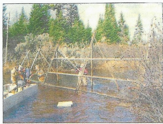
A fence is installed to prevent smallmouth bass from getting into Miramichi Lake.
